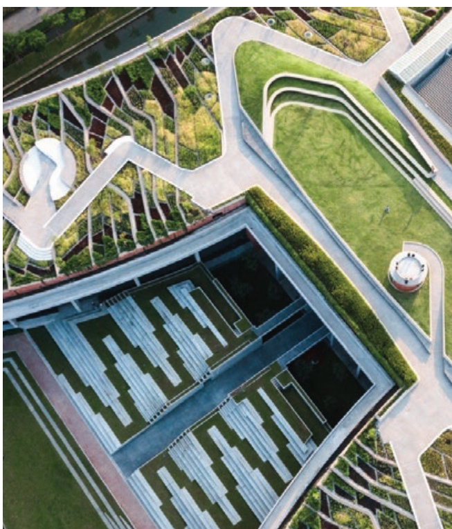
Repurposing 236,806 square feet of rooftop space, Thammasat University Rooftop is designed to mimic the structure of rice terraces for urban agriculture. Image: Landprocess
